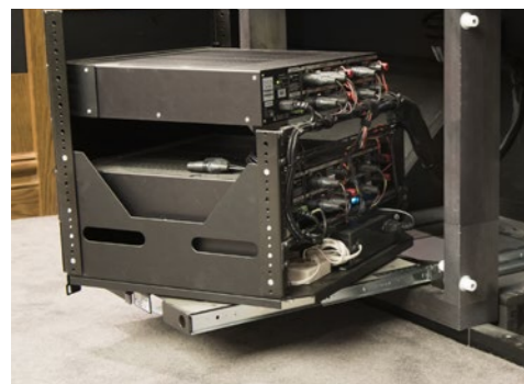
While the main equipment rack is outside the cinema room to minimise noise, light and heat, the Pro Audio Technology amplifiers for the front speakers and subs are at the front of the room, in the small rack shown above. “The reason is that we use balanced XLR cables to allow the signal to travel long distances with no loss,” says David Moseley. “But speaker cable works best when the cables are as short as possible. The surround channels are just as close to the rear rack, so we put the amps there for those speakers.”
